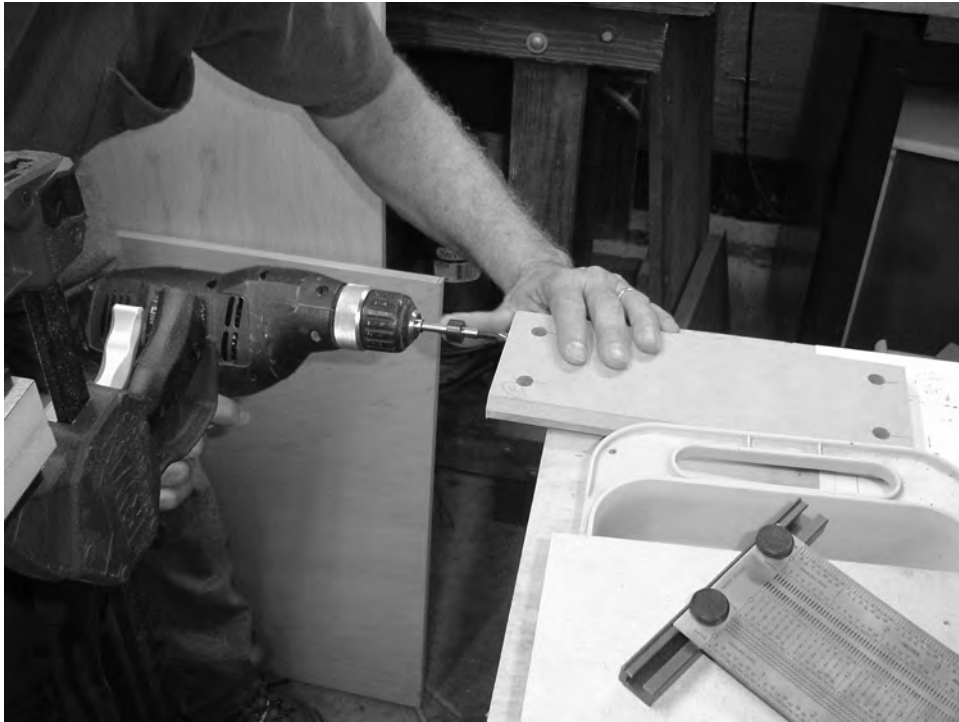
Figure 15-3. Drilling the 1/4" holes into the sides of Part F
