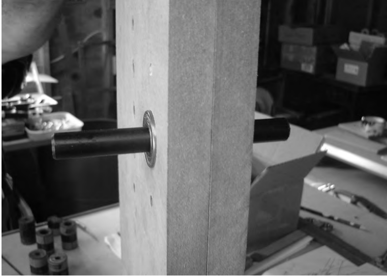
Figure 10-8. A 1/2" rod inserted to check that the 1 1/8" holes are lined up properly
